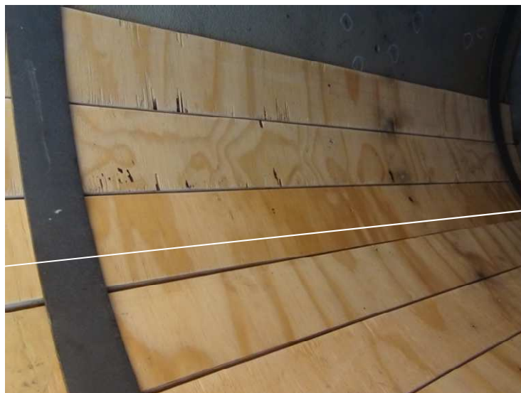
Figure 17: Exposed surface of Shutter board material to fragments and blast, along the length of the chamber.
