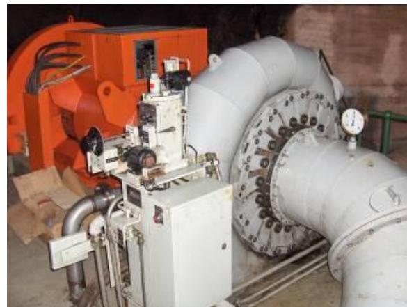
Figure 3 Powerhouse of the Mantsony'ane hydropower plant in Lesotho
