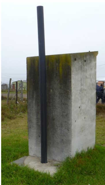
Figure 2 Cement Rocla structure in Goven Mbeki
