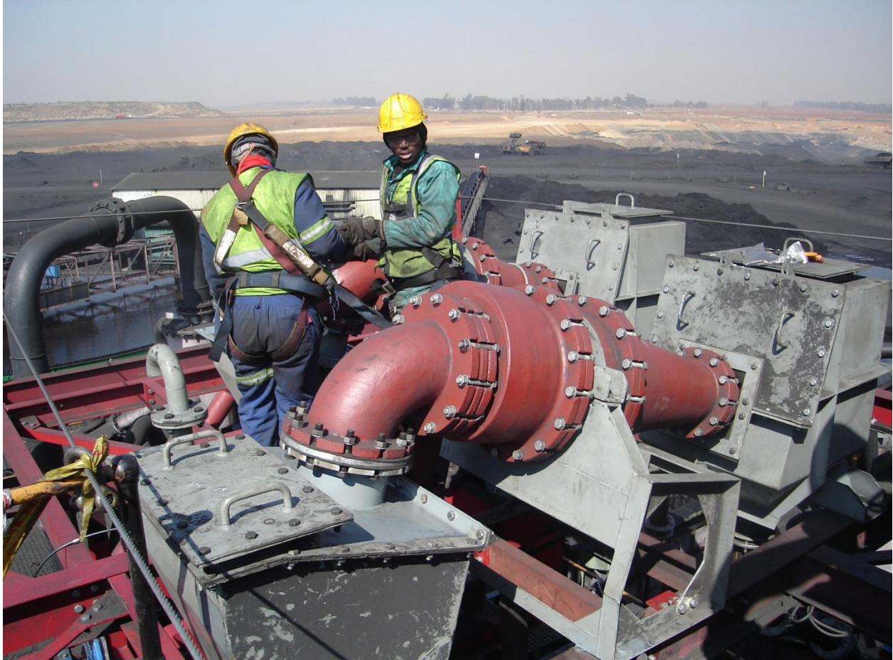
Figure 6. Dense-medium cyclones in Leeuwpan fine coal plant
