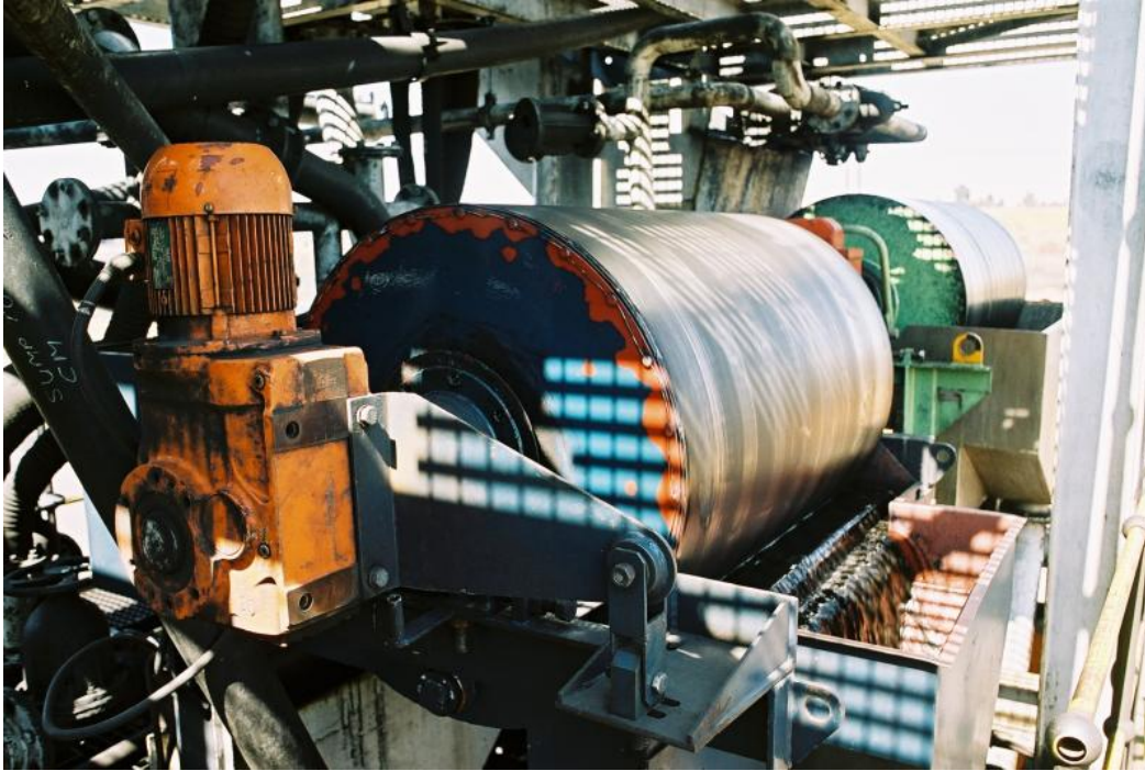
Figure 8. Magnetic separators in Coaltech pilot plant
