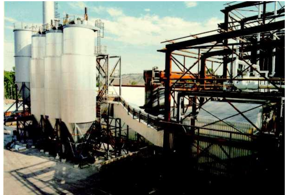
View of plant
