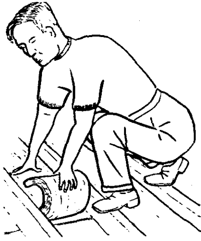
Laying insulation in the roof space.
