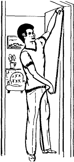
Draught proofing a door frame with self-adhesive strip.
