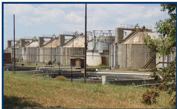
Conventional anaerobic digestion technology
