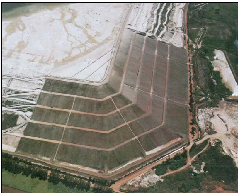
Figure 6: Rehabilitation of Daggafontein gold tailings dam (from AngloGold Ashanti, 2005)
