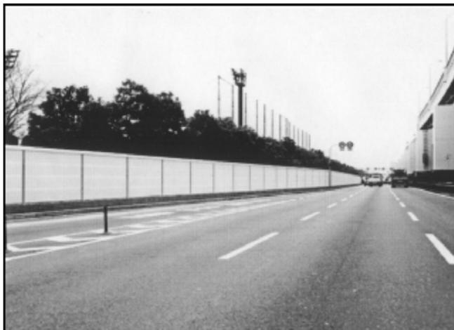
**Figure 1. View of soundproof highway walls coated with titanium oxide photocatalysts for the elimination of NO<sub>x</sub>. These new walls were constructed in Osaka, April 1999. (Anpo, M, 2000)**
