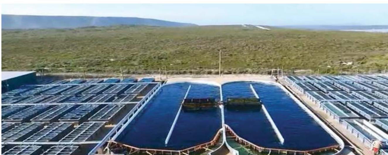
The Buffeljags abalone IMTA system, with ulva (seaweed) raceways in the center and the abalone tanks on the sides
