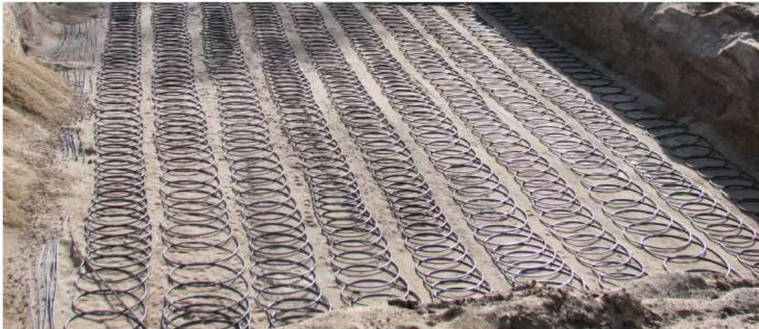
Figure 2: Layout of spiral earth coil (Lutchman 2018)
