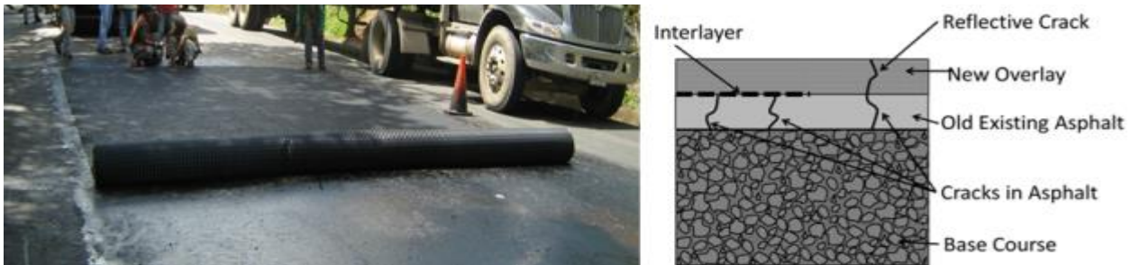
15 FIGURE 2 Geogrid Interlayer Reinforcement and HMA Overlay Construction.
