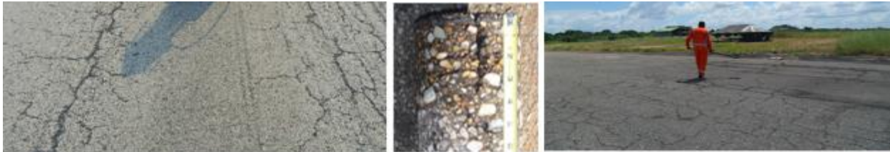
12 FIGURE 1 Example of an Old Cracked HMA Pavement.
