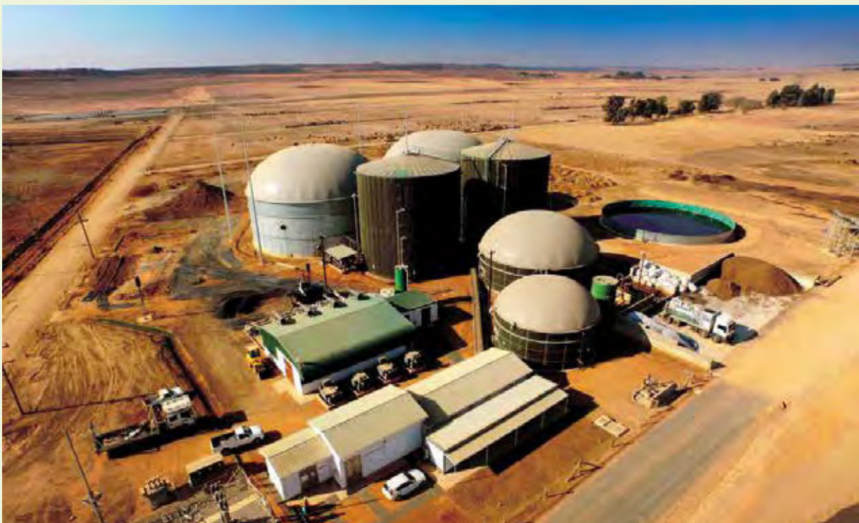
Bio2Watt biogas plant, Bronkhorstpruit
