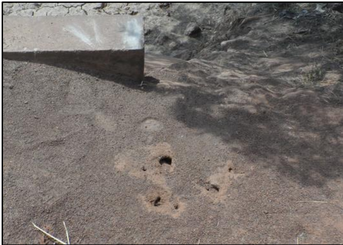
Fig. 2. Example of ant holes undermining the structural integrity of an embankment
