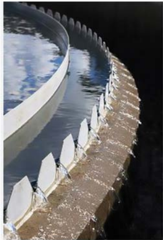
Figure 6.4: Image of sawtooth weir (Credit: Getty Images)
