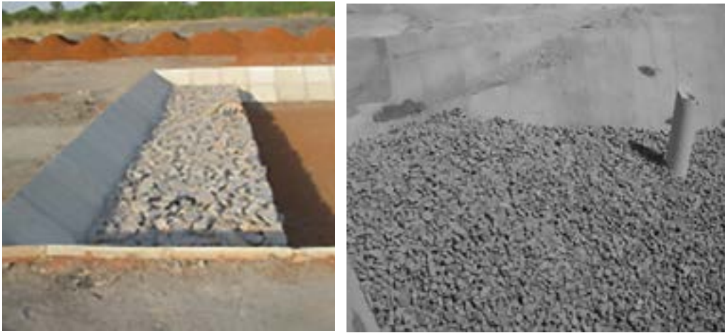
(a) The recommended arrangement. (b) Too fine materials used at the inlet/outlet.
