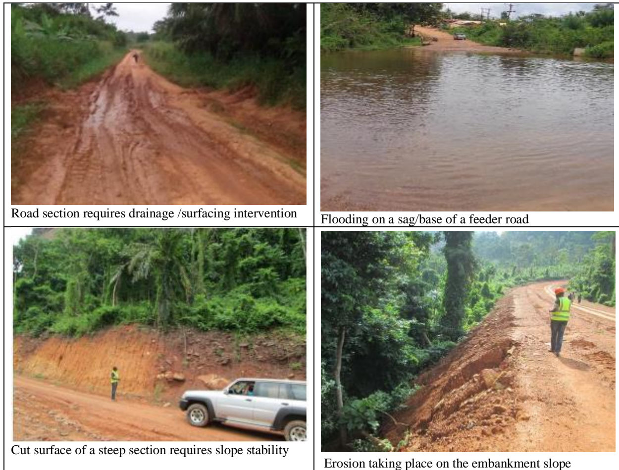
Figure 1: Some problems associated with steep slope gravel roads in Ghana
