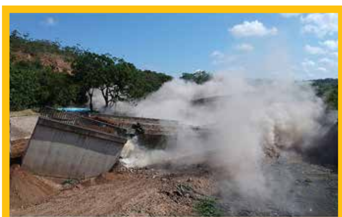
FIGURE 8: The demolition process was designed to minimise environmental effects
