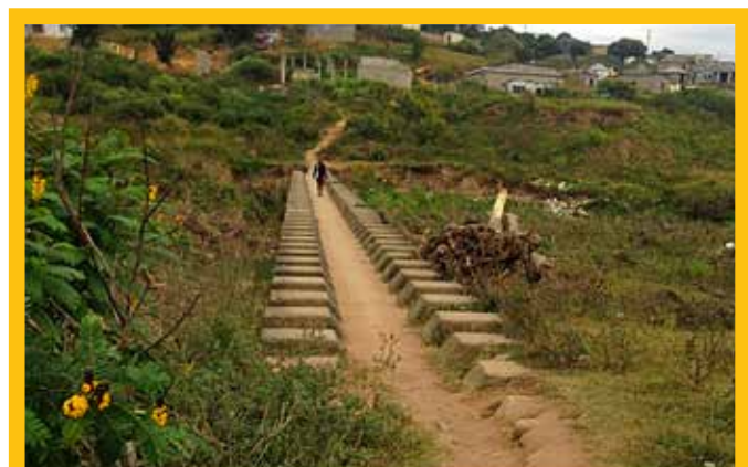
FIGURE 1b: The existing bridge prior to re-construction
