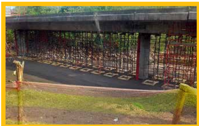
FIGURE 7: Sacrificial props maintained stability until demolition
