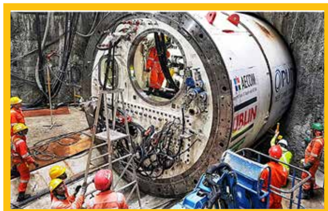
FIGURE 5: TBM with cutter head removed
