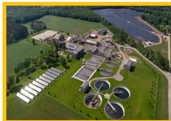
FIGURE 4: St. Cloud Wastewater Treatment Facility, Minnesota, USA 23
