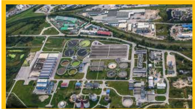
FIGURE 7: Hiller Park Wastewater Treatment Plant 27
