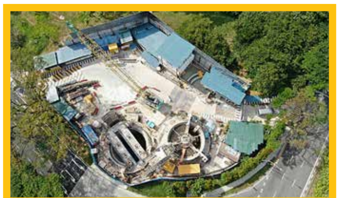
FIGURE 9: Aerial view of shaft sinking site
