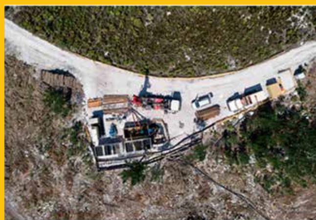
FIGURE 5: Production borehole drilling in progress showing sumps (a series of containers) and temporary pipelines
