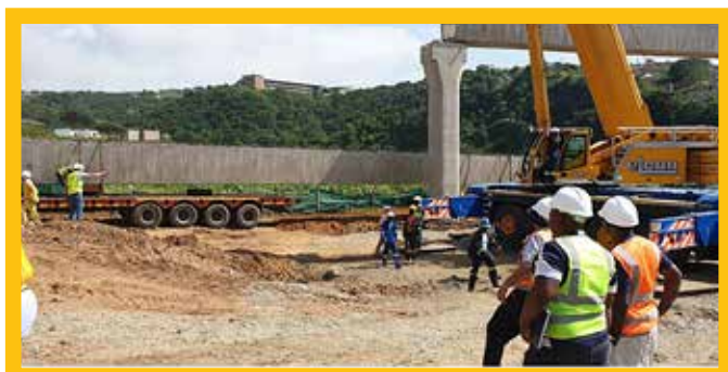
FIGURE 4: Installation of bridge decking
