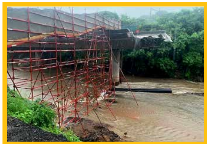
FIGURE 10: Temporary supports had to withstand repeated flooding
