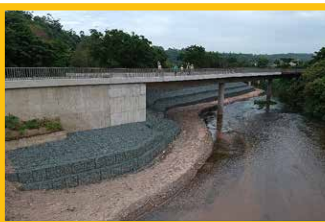
FIGURE 11: The new abutment is unusually heavy and sits behind extensive protection works
