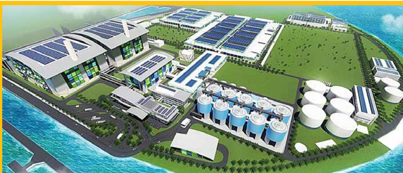
FIGURE 10: Tuas Water Reclamation Plant
