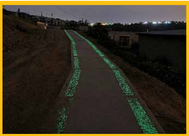
FIGURE 8: Illuminating sidewalks leading to the bridge
