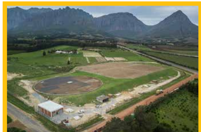
FIGURE 9: Completed Leliefontein PAT station in foreground, with 36 Mℓ and 100 Mℓ reservoirs in background
