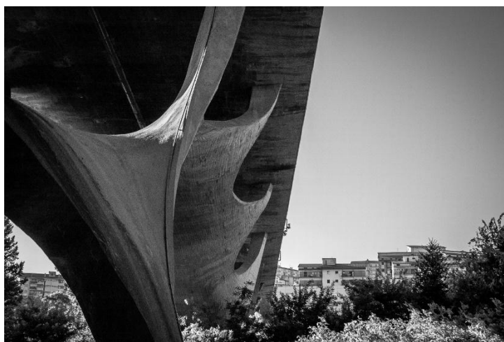
Figure 2: Basento river bridge (Luongo, 2016)
