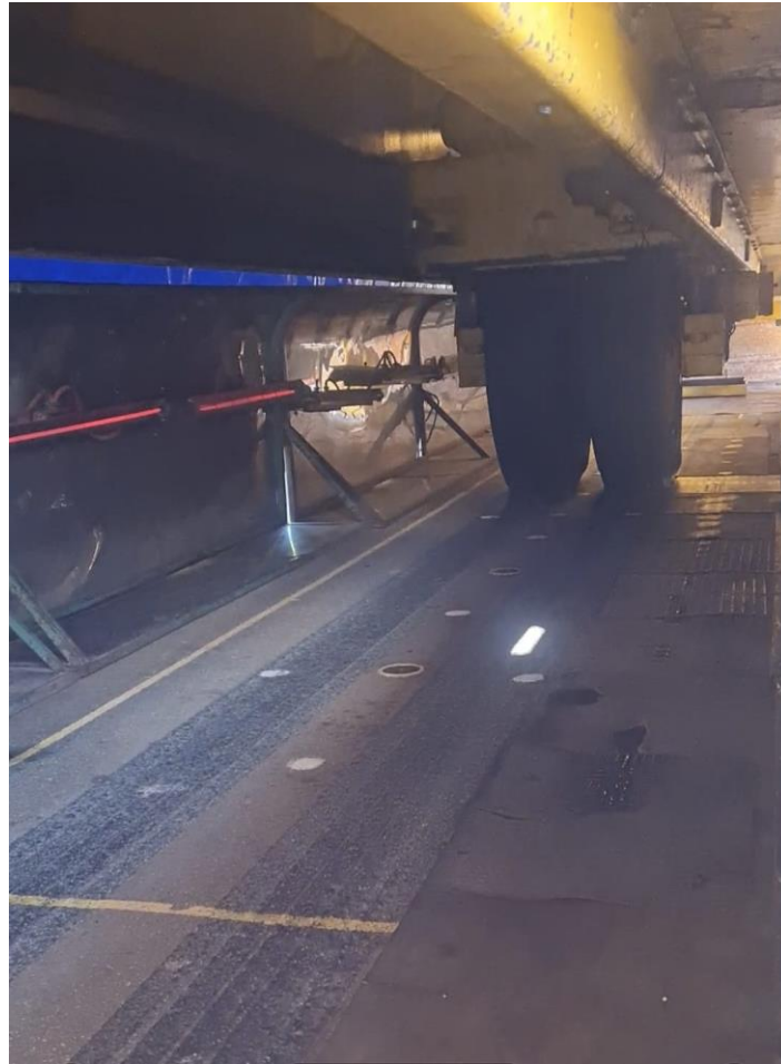
Figure 5: Heater set up on the HVS section.
