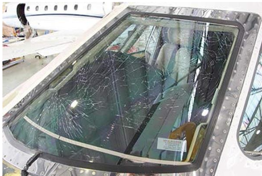
Hail damage to cockpit window
