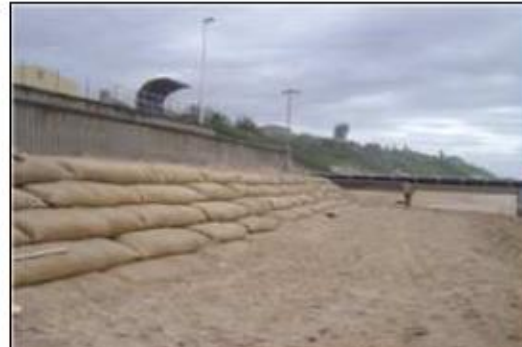
C11 Geotextile shore protection in low to moderate wave energy environments
