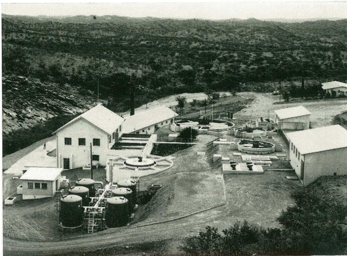
The integrated water reclamation and water purification plant at Windhoek. The reclamation process was developed jointly by the NIWR and the Windhoek Municipality
