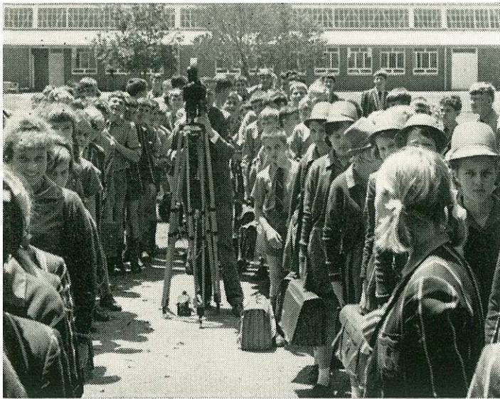
Filming during the production of "The Buildings In Your Life", the latest film in the CSIR series 'Science In Your Service'. The location is a CSIR-designed high school near Pretoria
