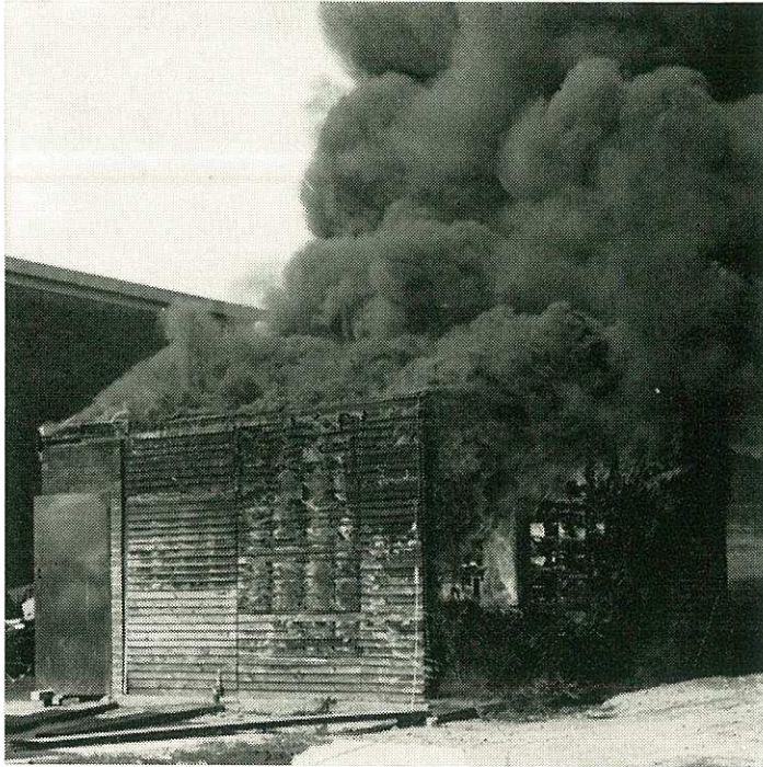
Burn-out test in progress on a light-weight form of house construction
