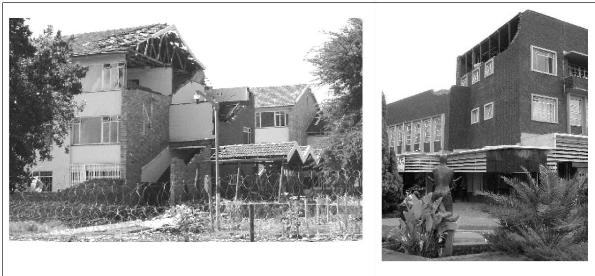
Figure 3. Buildings in Stilfontein damaged by a M_L =5.3 tremor on 9 March 2005 (photograph R.J. Durrheim)
