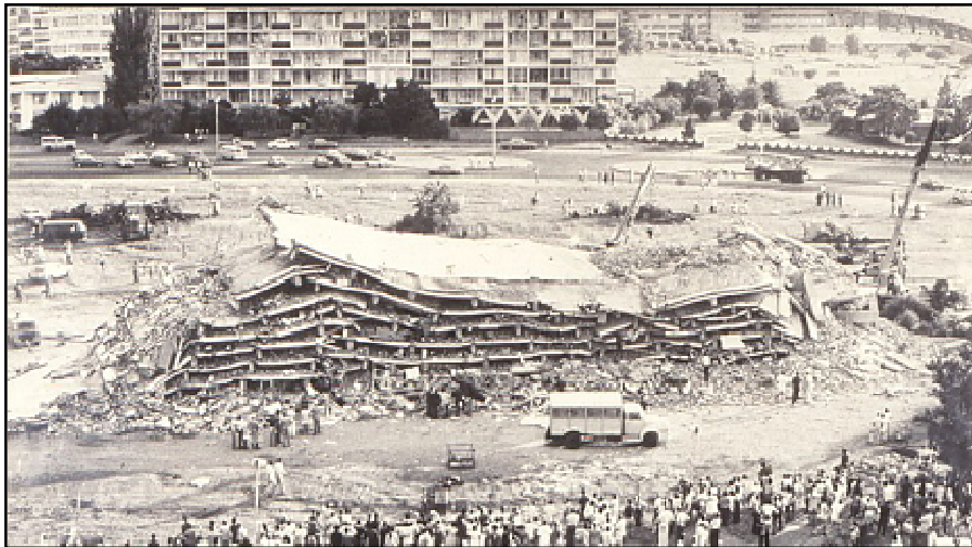
Figure 8. Apartment block in Welkom that collapsed following an M_L=5.2 tremor on 8 December 1976 (The Star)
