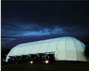
UMkhanyakude Pavilion structure sponsored by Siemens
