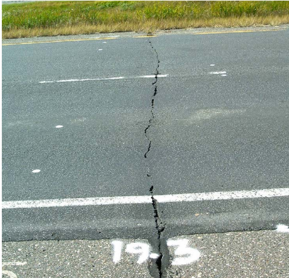
FIGURE 2 Reflected transverse crack through the slurry seal .
