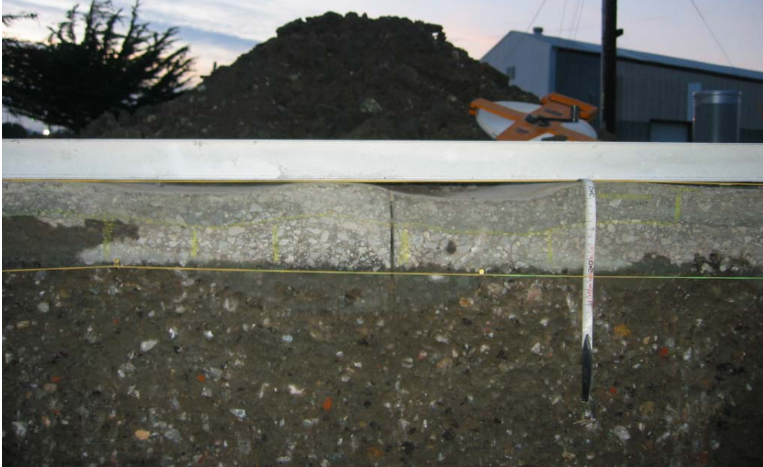
FIGURE 10 Test pit face showing rutting pattern on 45-mm MAC15 and 90-mm DGAC.
