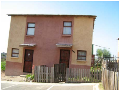
Figure 3. Semi-detached double storey unit.
