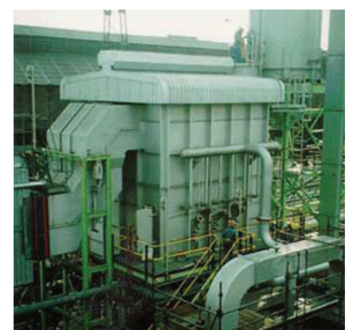
High Sulphur Pitch Incinerator
