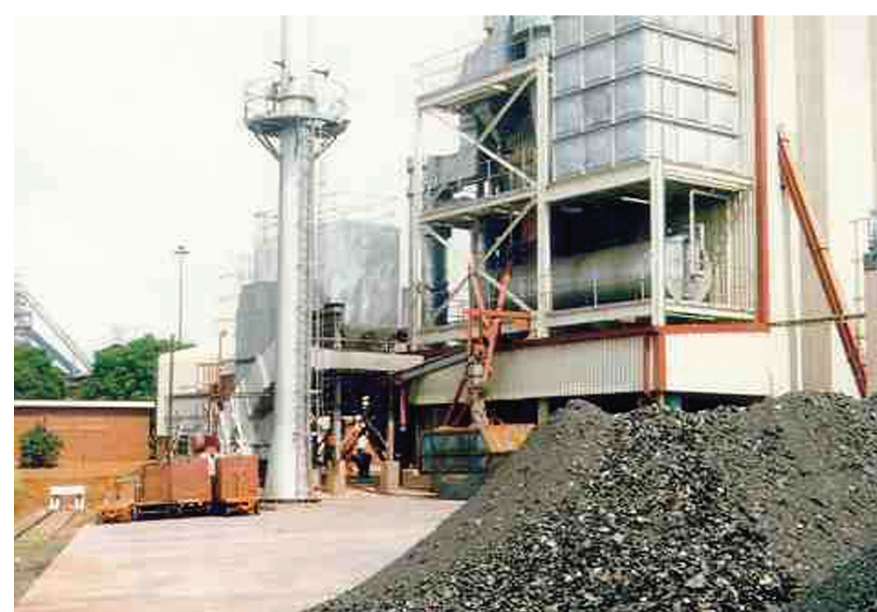
1984: National Fluidised Bed Combustion Boiler
