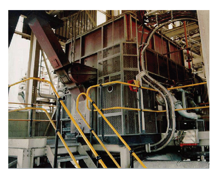
Hot Gas Generators
