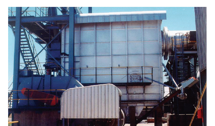
Slagment Hot Gas Generator
