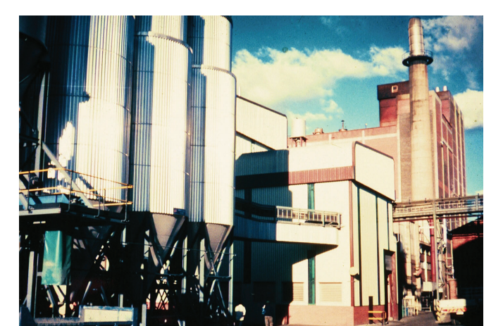
Biomass Sludge Boiler
