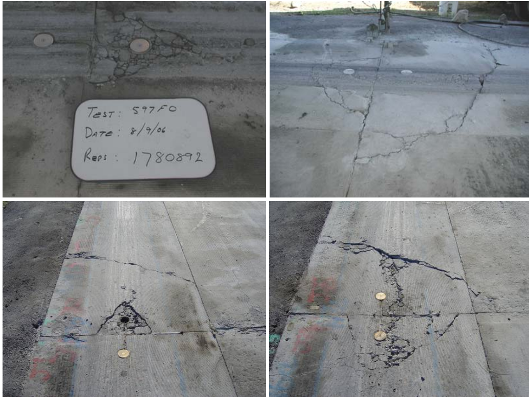
Figure 11. Transverse and longitudinal view of the two failed joints at the end of pavement life in Section 1
