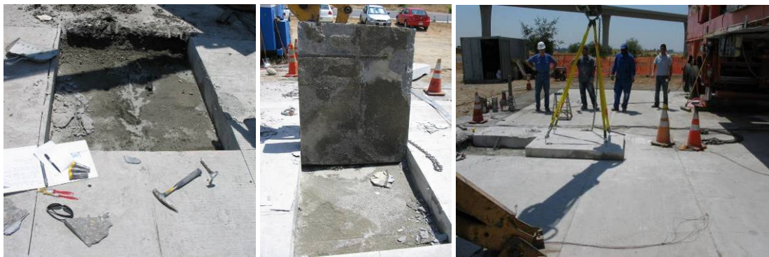
Figure 12. Investigation of void under the slab in Section 2
