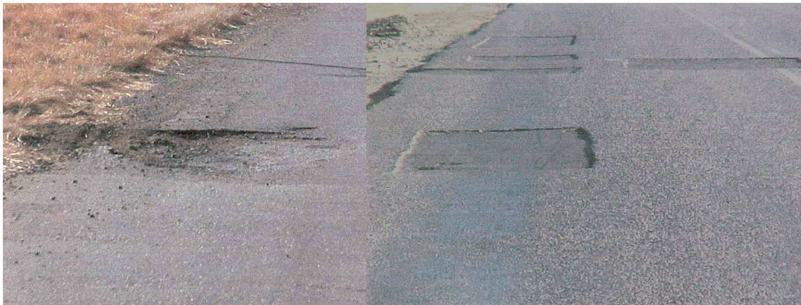
Figure 6: Potholes and unevenness causing tyre impact damage and heat build-up.
