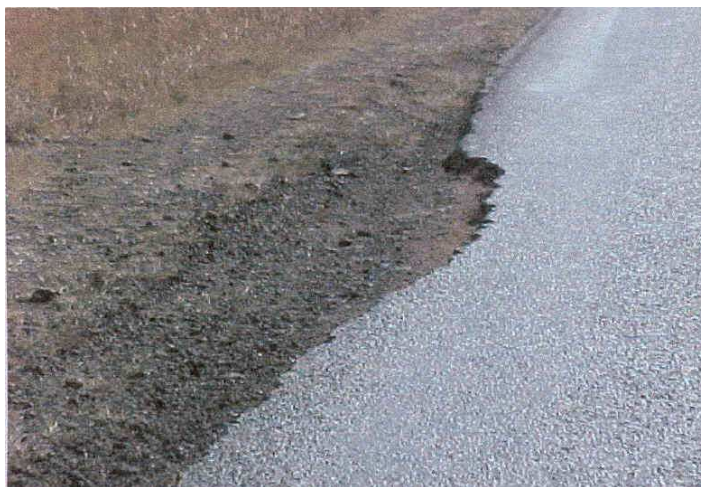
Figure 7: Edge break causing tyre impact damage and heat build-up.
