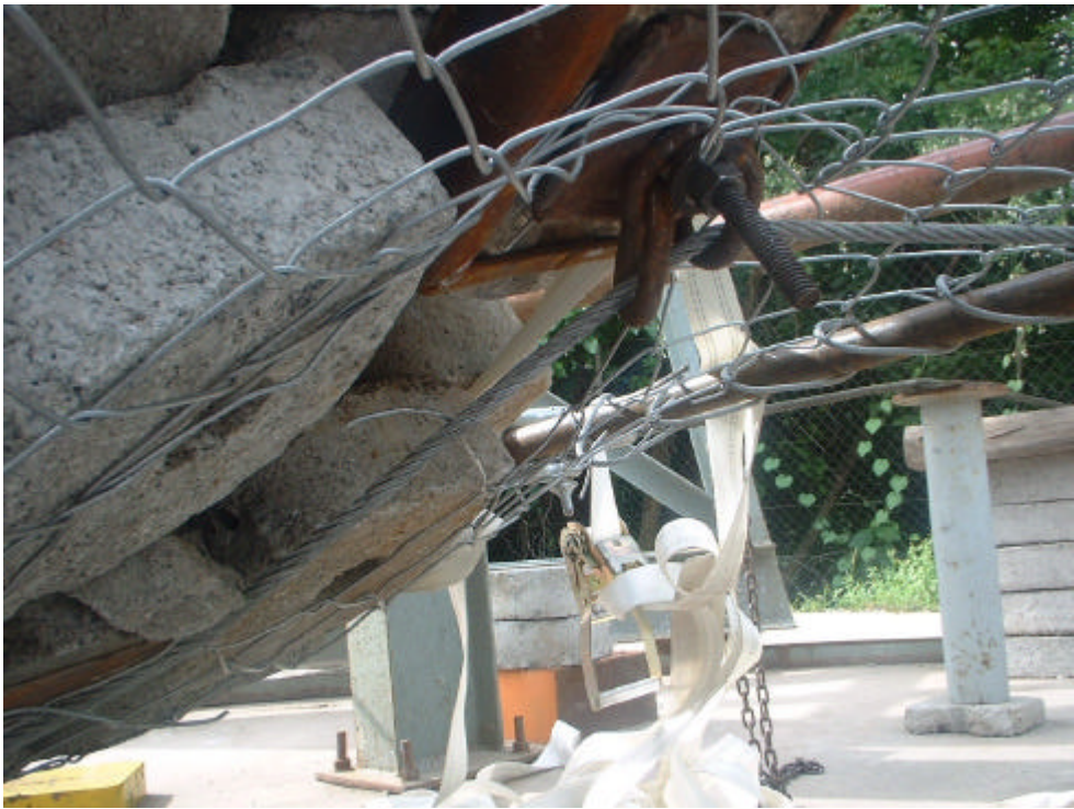
Figure A-43 Localised mesh damage around a bearing plate in the test on 29/01/02
