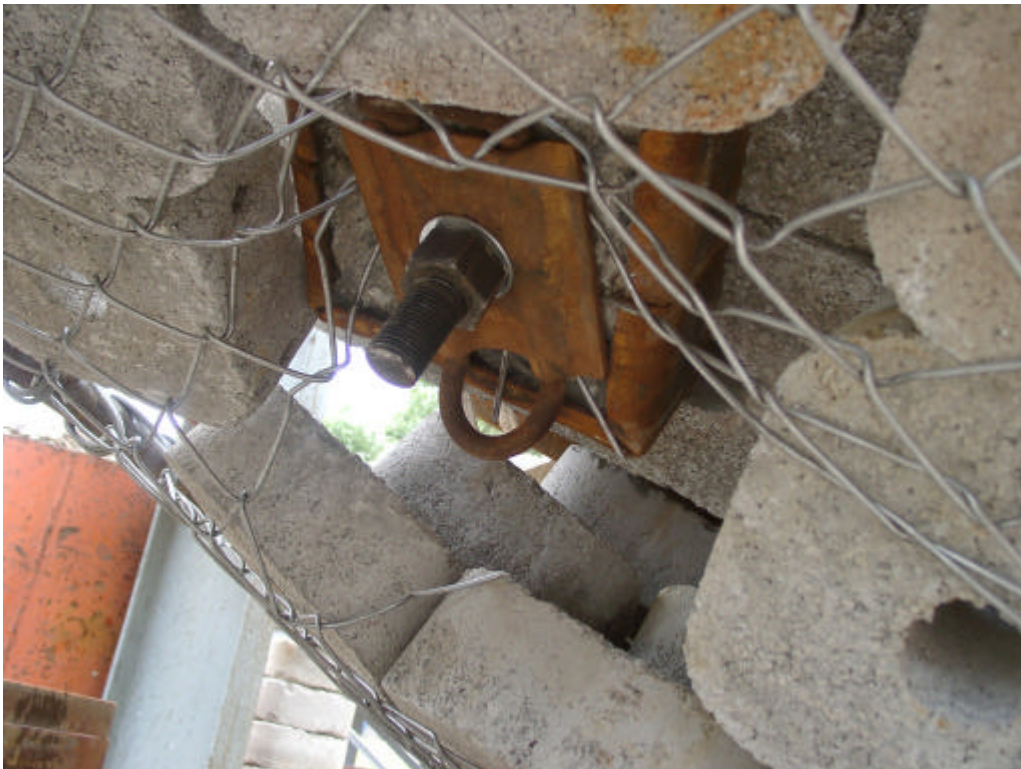
Figure A-13 Bending of bolts in test 19/11/01
