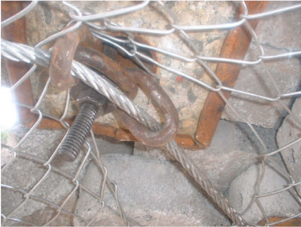
Figure A-40 Localised mesh damage around tendons in the test on 23/01/02
