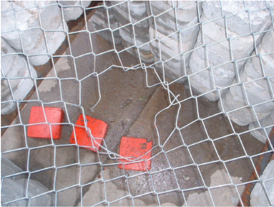
Figure A-22 Failure in the test on 21/01/02
