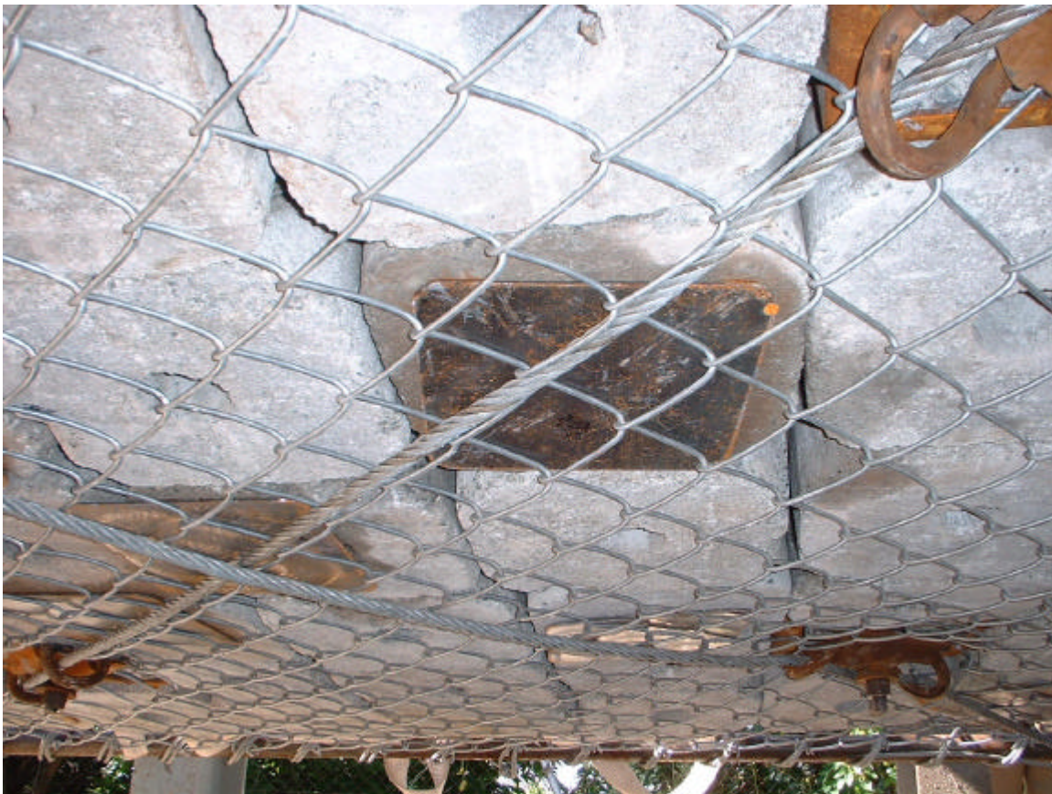
Figure A-1 Lacing and diamond mesh used in the test on 30/10/01
