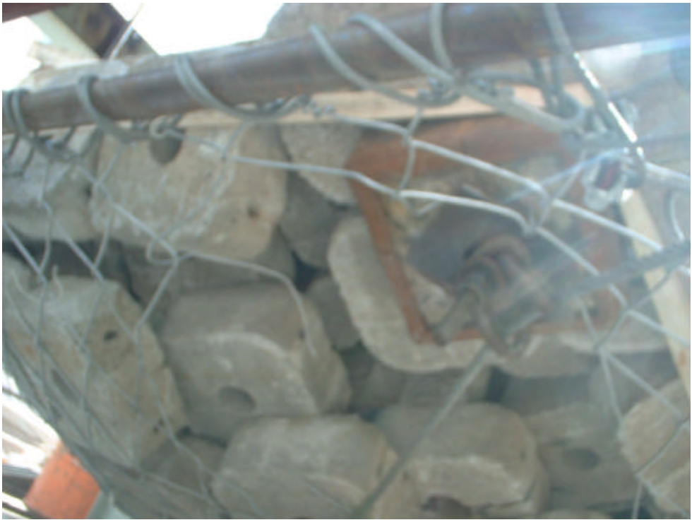
Figure A-56 Localised mesh damage around the bearing plates in the test on 25/02/02
