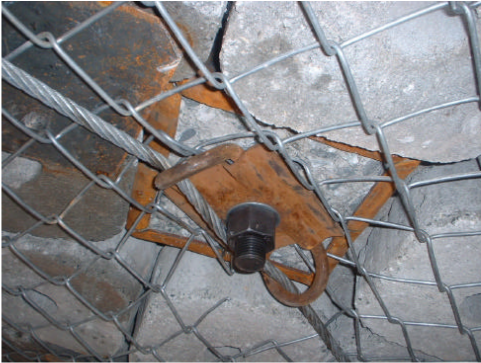
Figure A-8 Localised mesh failure near the tendon
