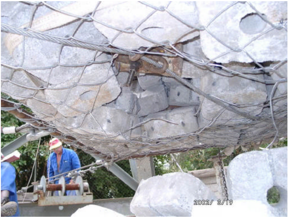
Figure A-63 Mesh damage around bearing plate in the test on 19/03/02
