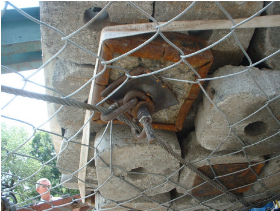
Figure A-53 Mesh damage around the bearing plate in the test on 19/02/02
