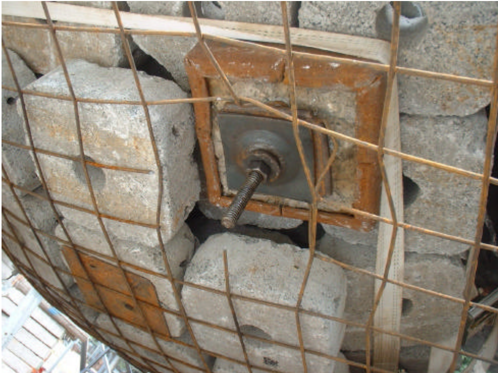
Figure A-50 Localised mesh damage around a bearing plate in the test on 07/02/02
