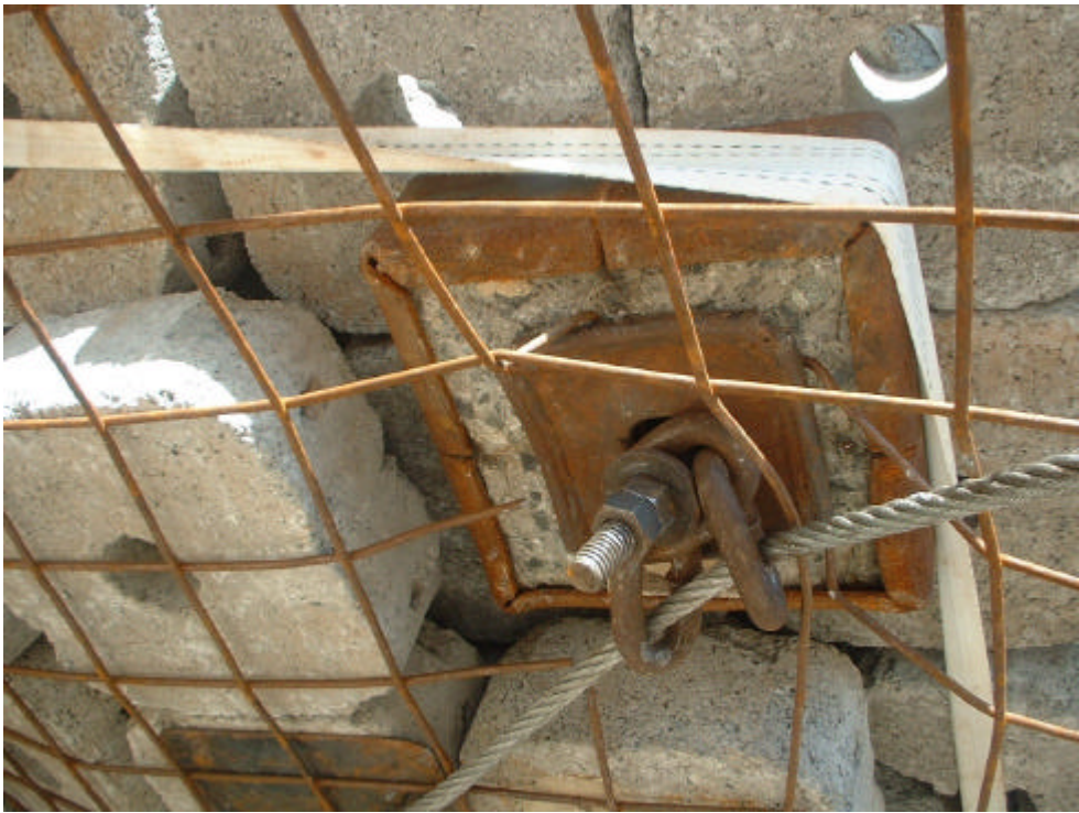
Figure A-45 Limited mesh damage around a bearing plate in the test on 02/02/02
