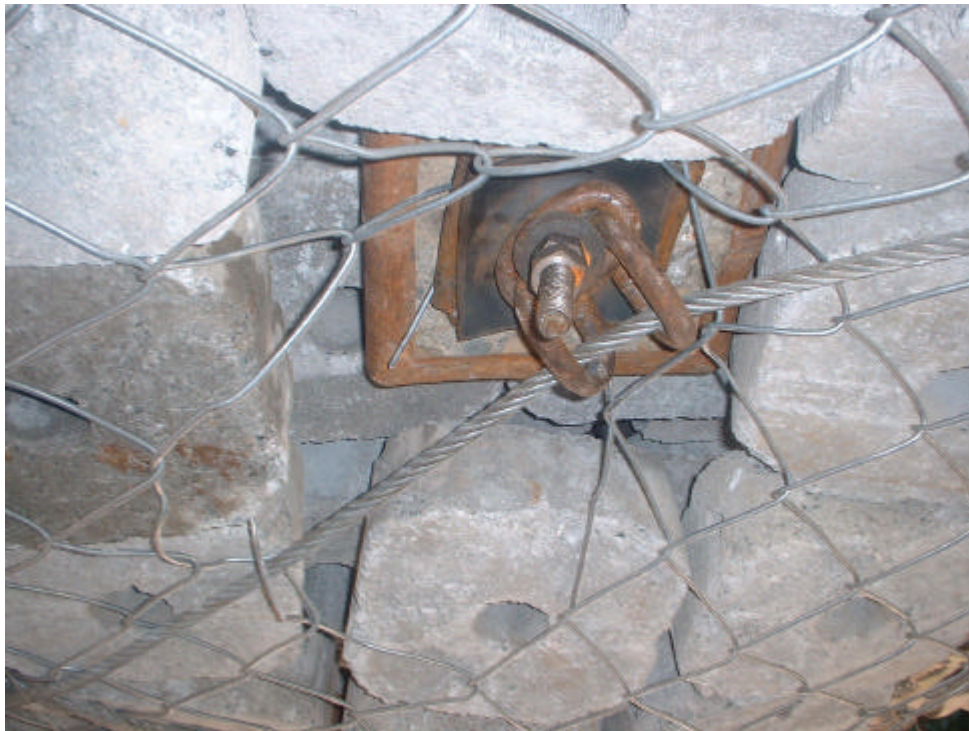
Figure A-66 Local mesh damage around lacing and tendon in the test on 22/03/02
