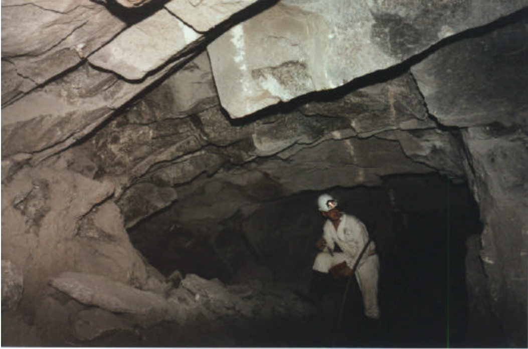
Figure 3.9 - Prominent jointing causing unstable conditions over a Merensky reef stope gully. An additional support pillar has been left on the up dip side of the gully, on the right of the picture.
