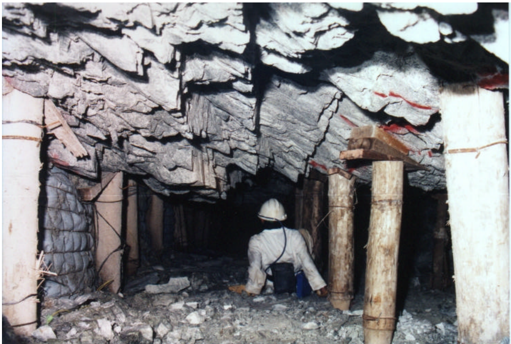
Figure 3.4 - Blocky hangingwall conditions arising from the interaction of jointing and stress induced fracturing when mining West on the Carbon Leader Reef at approximately 3400 m depth. In this instance in-stope ground control of these conditions is good.
