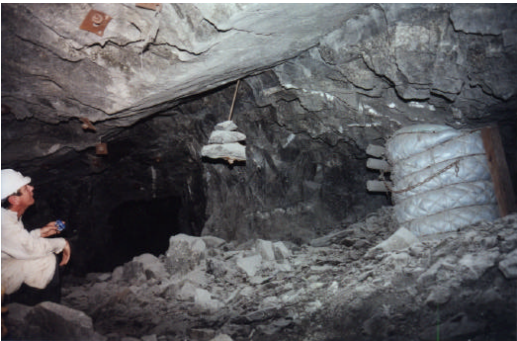
Figure 3.10 - Fall of ground associated with flat dipping sill on Merensky reef at 1800 m depth. Bolting failed to prevent falls in gully; RSS packs captured brow and prevented migration of fall into panel.
