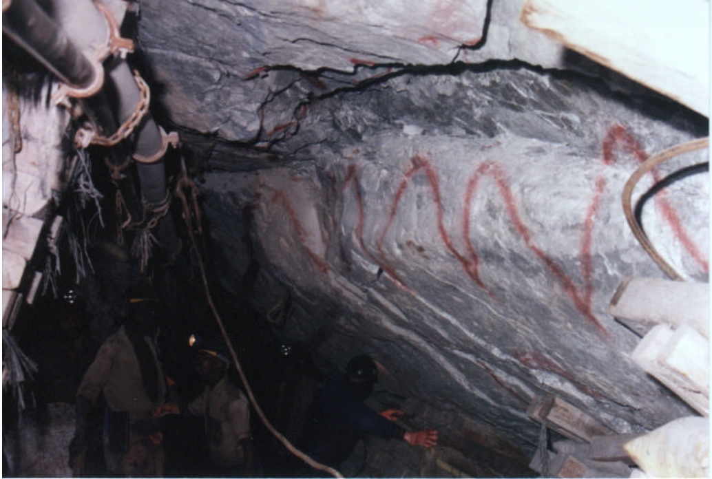
Figure 3.5. - Typical brow on Basal reef where shear parting rolls sharply upwards into the hangingwall. Rock is loose on the up-dip side of the marked brow (to the left), while the brow on the parting is generally stable.
