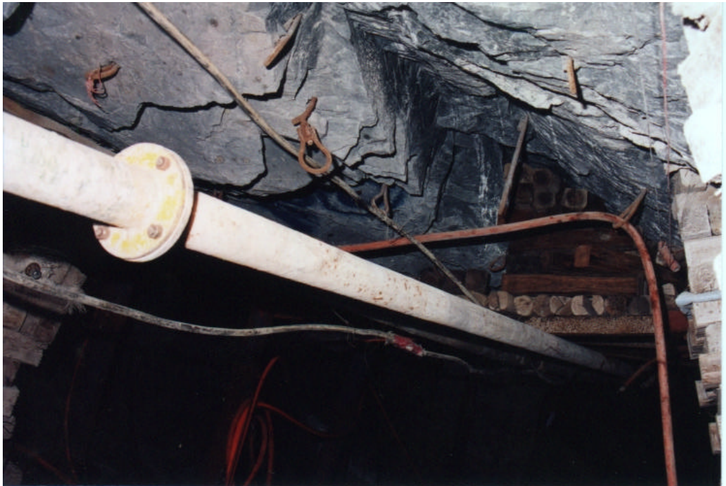
Figure 3.2: Typical joint-bound fall of ground along a reef drive on the VCR.
