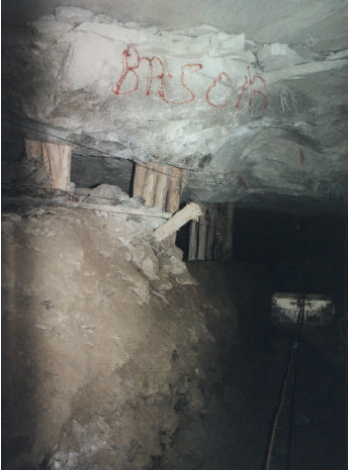
Figure 3.11 - 2.5 m high brow created by partial collapse of a dome on the Merensky reef. Controlled by stiff elongates cluster
