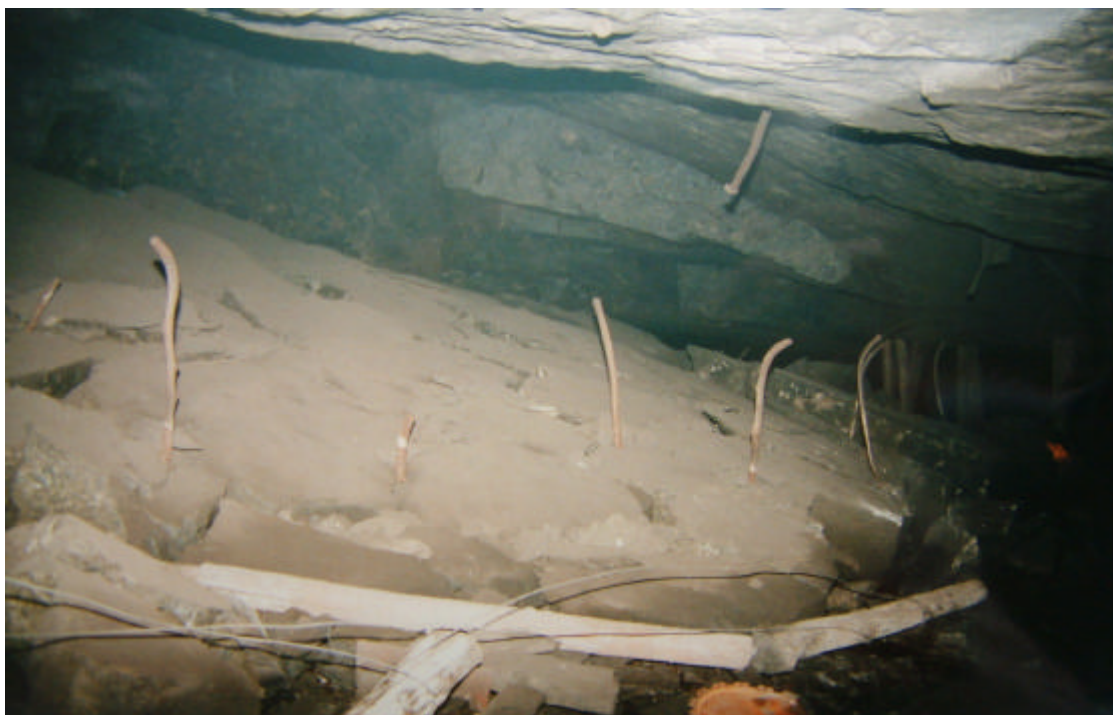
Figure 3.14 - Collapse of a major dome in a platinum mine at shallow depth: installed rebar bolts proved inadequate to support the large wedge of ground. In this example the wedge is approximately 50 m long, 8 m wide and up to 4 m high. The sketch, top, explains the mechanism.
