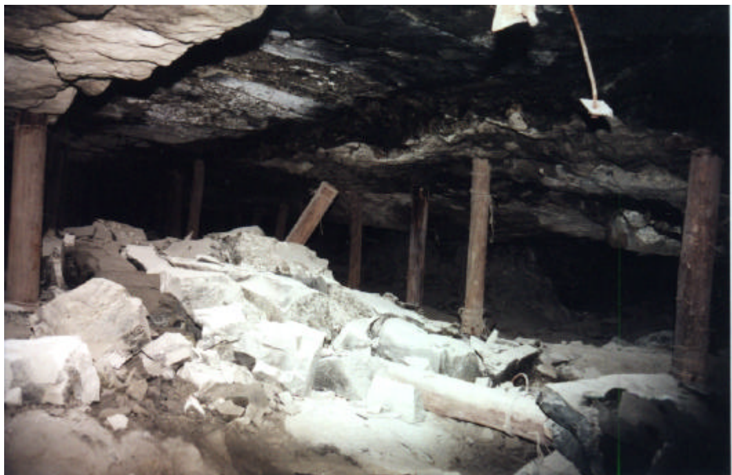
Figure 3.8 - Collapse of 0.5 m to 1 m of hangingwall within a 1.5 m wide dyke in a Merensky reef stope. Additional support is placed along the dyke contacts, but not beneath the dyke.
