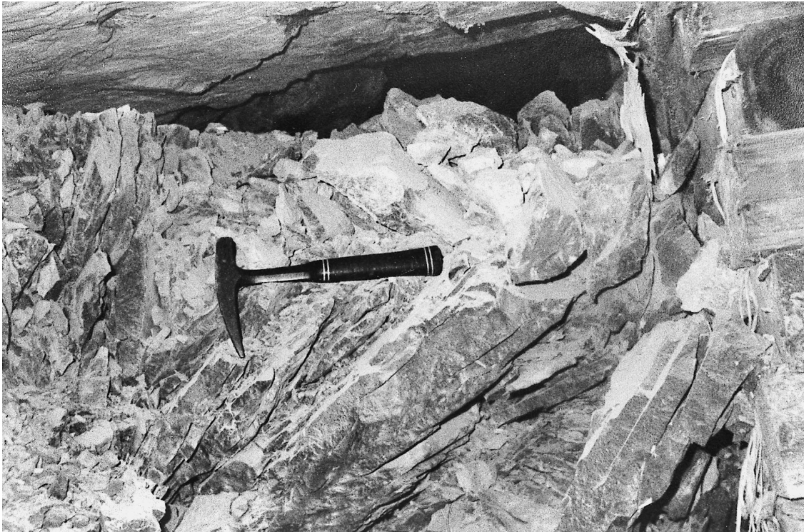
Fig. 7. Rock ejected from the footwall and face between F and G (Fig. 6) into the space between the original face position and the first dip line of packs. The photograph is taken looking updip with the face to the left. Note the intact hangingwall.
