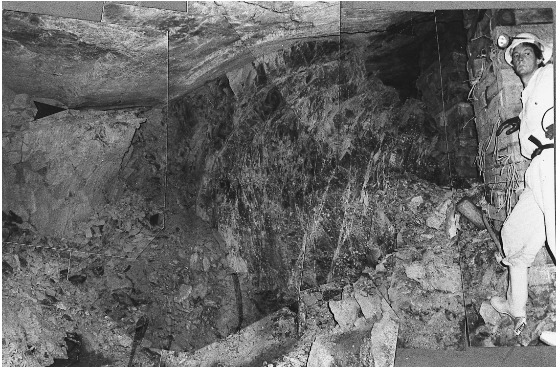
Fig. 8. Photo mosaic showing the up-dip face where the fatalities occurred, viewed from position H (Fig. 6) and looking up-dip. The timber packs on the right are situated to the east of the roll. The hangingwall fragmented during the rockburst. Most of the fallen rock was subsequently removed. Note the numerous fractures and joints in the face, and the smooth surface marking the parting above the collapsed brow.
