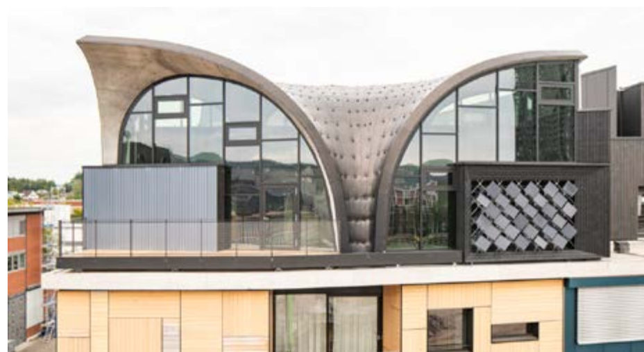
HiLo - Research & innovation unit for NEST, Dübendorf, Switzerland, 2011-2021: This research demonstrated the structure for an unreinforced concrete floor consisting of a thin funicular vault stiffened by a series of spandrel walls on its extrados. A first version of this innovation is built in the NEST HiLo project, realized in 2021 on the Empa campus in Dübendorf, Switzerland.
