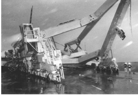
Fig. 13. Collapse of container crane.
