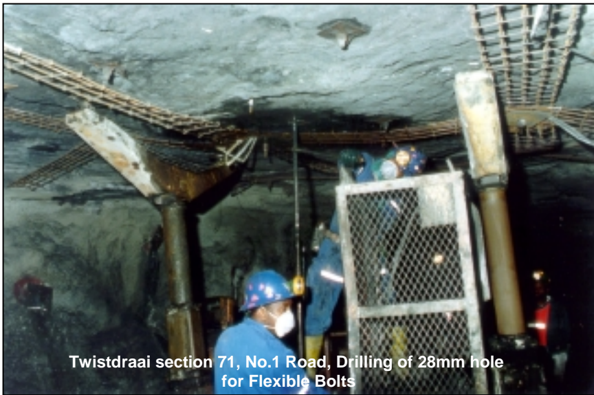
Twistdraai section 71, No.1 Road, Drilling of 28mm, for Flexible Bolts
