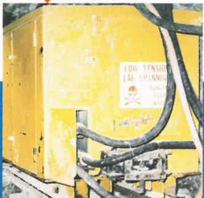
Mobile Miniature Sub Station 200kva
