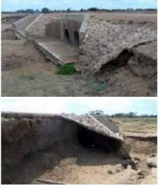
Figure 5 Damage to culverts and erosion protection.
