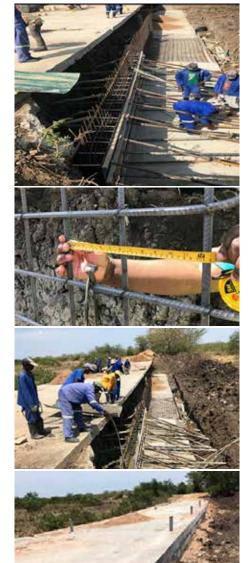
During the construction of the concrete wall, quality control tests were conducted on the concrete as well as on the gravel material used for backfilling. The material for the concrete consisted of aggregate with 19 mm Nominal Maximum Aggregate Size (NMAS), river sand, and a 42.5N cement class.
