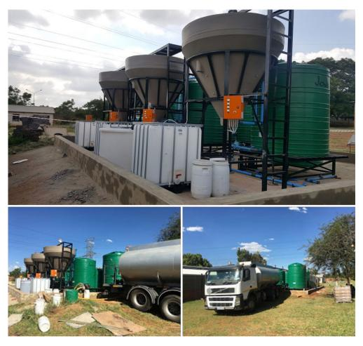
Figure 2. An illustration of the developed AMD treatment plant with the tanker loading AMD.
