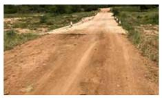
Figure 4 Damage to the road approaching concrete fords.
