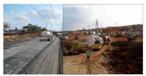
compaction of all layers of a new road with a G3 base course under a Cape seal surfacing. These experiments have shown that, provided certain precautions are taken in the design and construction, seawater can be used in all layers including a G3 base course without experiencing any significant degree or extent of salt damage, either during construction or in the long term – at least up to 36 years [8].
