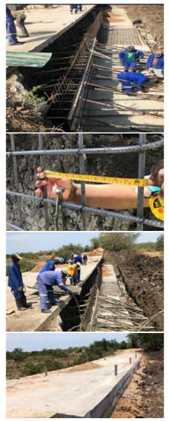
Figure 10 Construction of concrete wall.
