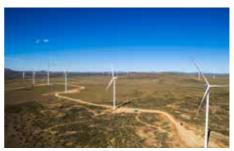
Noupoort Wind Farm consists of 35 turbines with a total output of 80MW. When operating at full capacity, it generates around 304 800MWh of clean renewable energy per year and is expected to supply electricity to power up to 91 835 South African homes.
