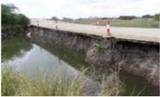
Figure 3 Erosion and undercutting of concrete fords.
