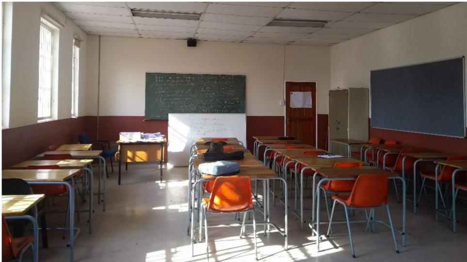
**Figure 5.** Photo of classroom at School D showing lack of sound absorbing objects and materials.
