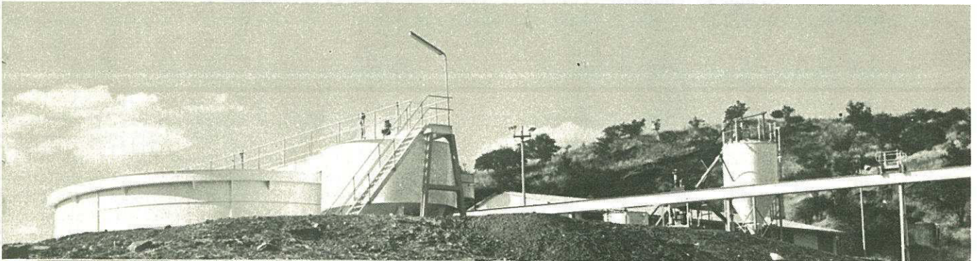
Windhoek water reclamation plant (p. 28): At this plant in Windhoek (top) purified sewage effluent is reclaimed for domestic use.
