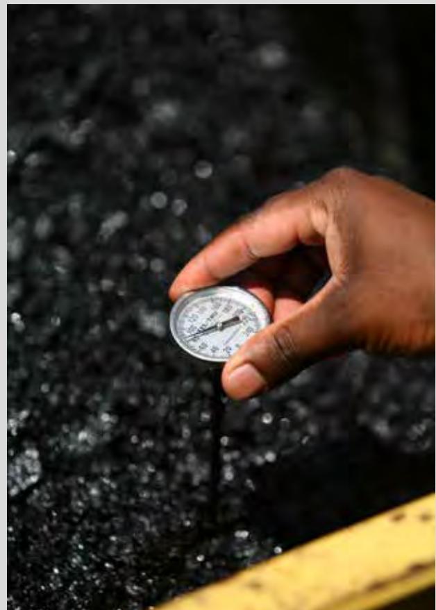
Measuring the temperature of asphalt.
