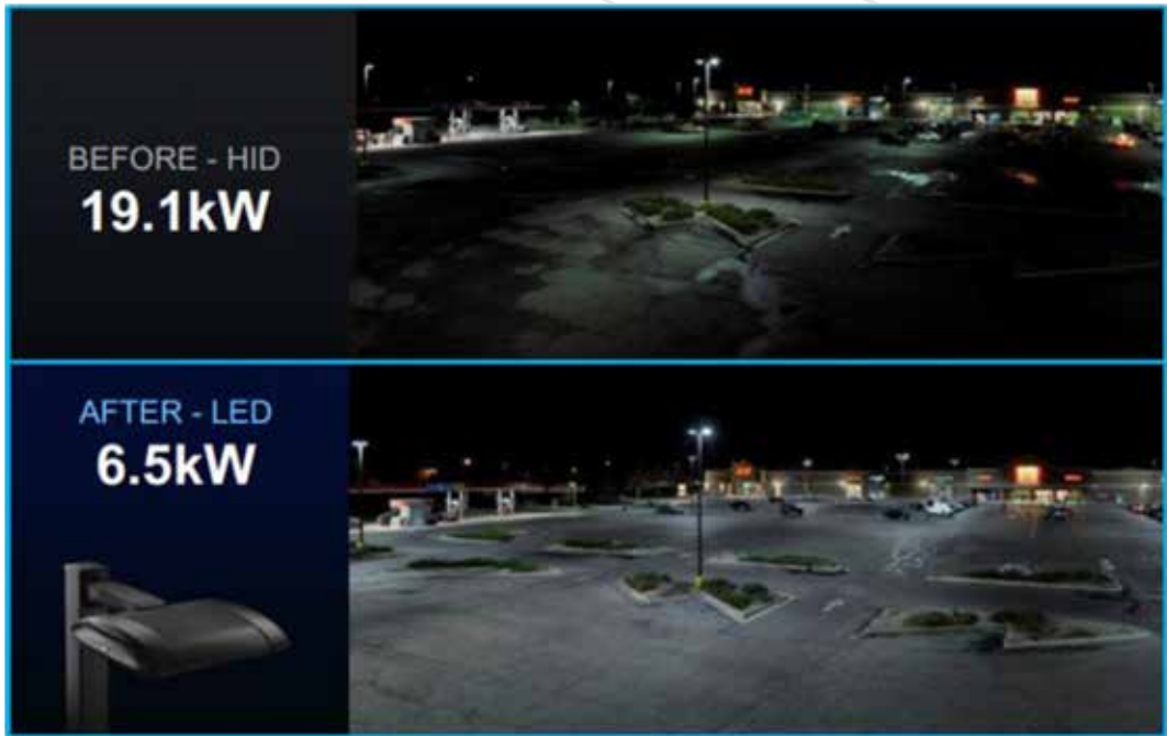
Figure 5-2: A parking lot of Edgewater marketplace (Colorado-USA) before and after lighting retrofit using LED fixtures (US DoE, 2016)
