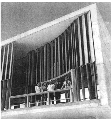
Figure 9: Oscar Niemeyer's use of brise-soleil at Belo Horizonte Yacht Club in 1940. (wikiarquitectura, 2010)
