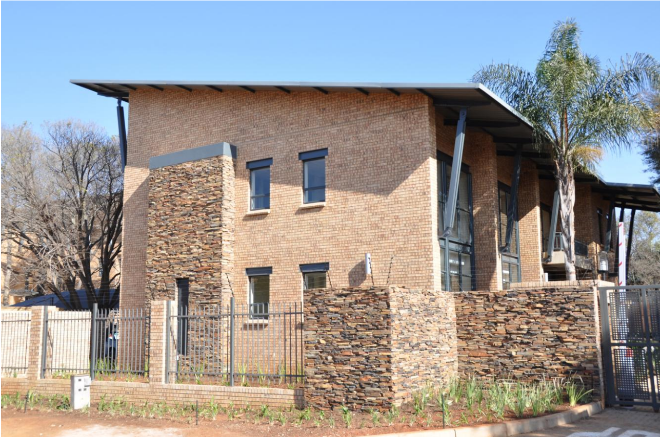
Figure 8: Typical office building being built within the last decade in Pretoria with good northern solar protection. (Author)
