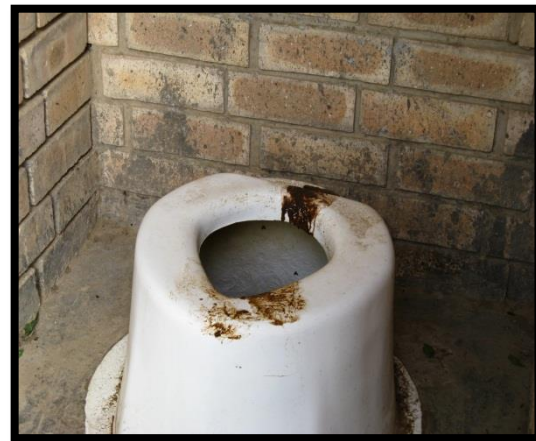
Figure 2 Serviceable school toilet facilities
