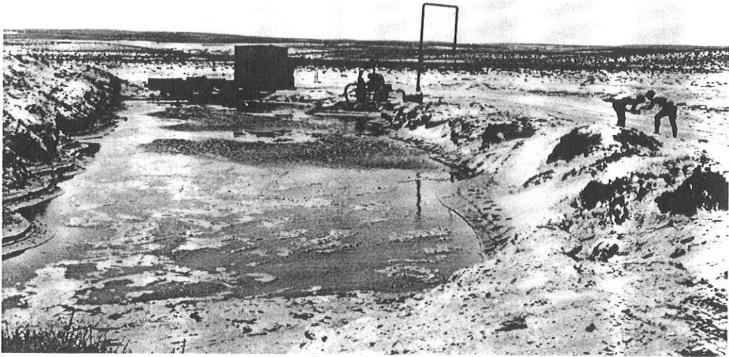
FIG. 3 : Eastern arm of excavated water trench in the riverbed at the mouth of the Holgat. The pumping equipment can be seen in the background. (ECRU 80-10-14)
