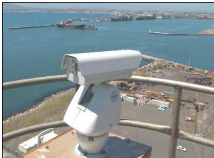
Figure 2: PTZ video camera on top of Port Control
