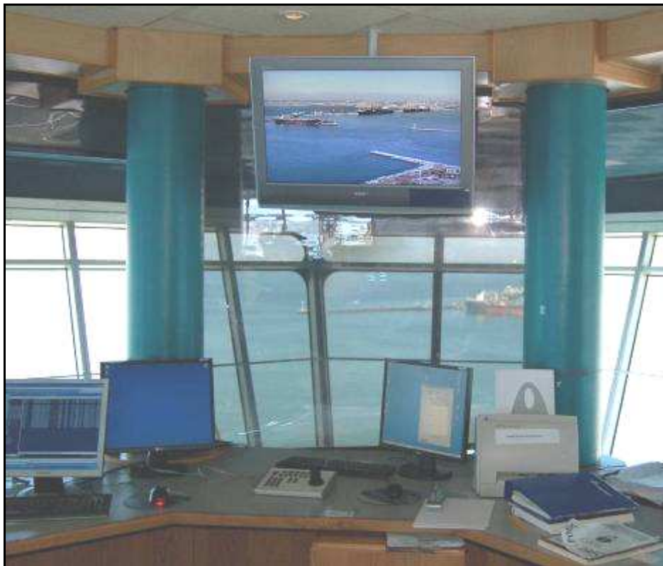
Figure 3: LCD Monitors and keyboard controller at Port Control
