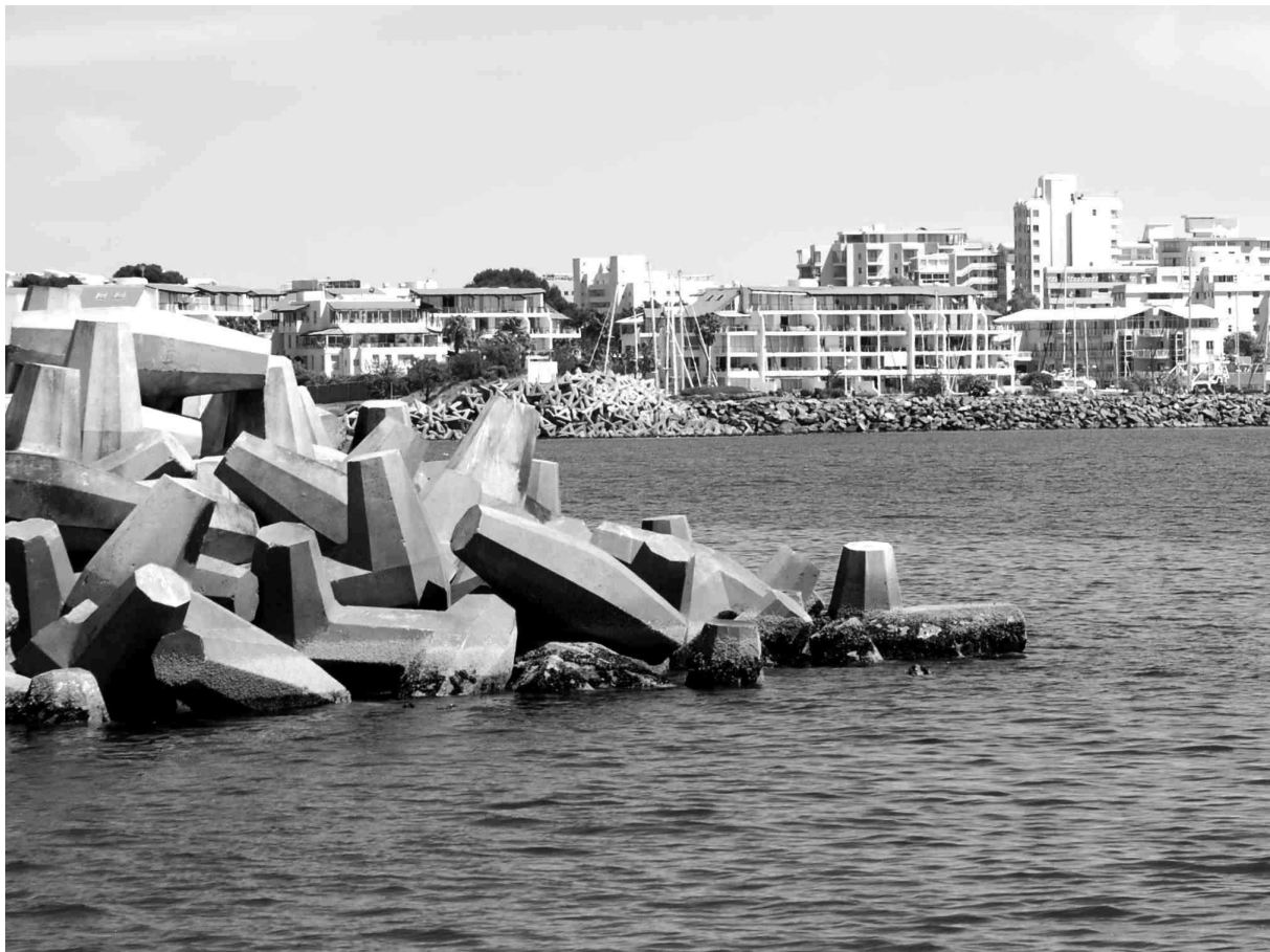
Figure 1: Dolosse protecting Cape Town's harbour
