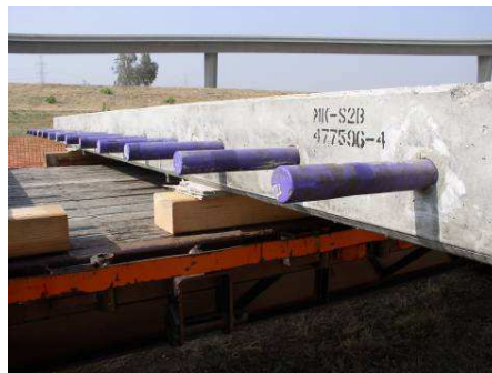
Figure 1. Precast Dowels and slots showing slot/dowel bar connection
