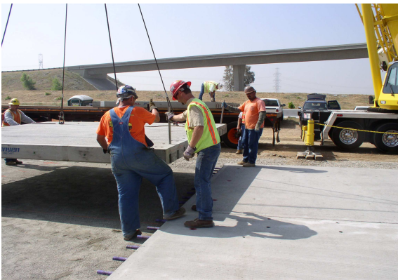
Figure 2: Slab positioning and core showing dovetail slot/dowel bar connection
