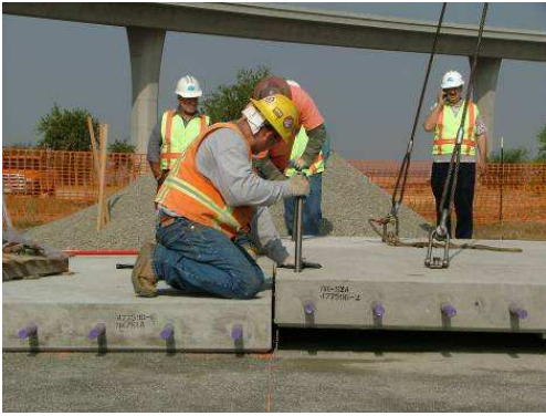
Figure 4. Precise placement of the slab on the sand bedding layer and hose with fitting for injecting grout
