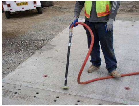
Figure 4. Precise placement of the slab on the sand bedding layer and hose with fitting for injecting grout
